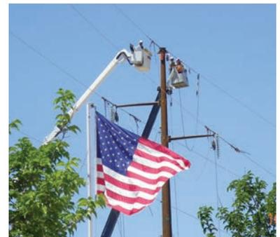
Conductor is installed on the Roswell Loop project.
