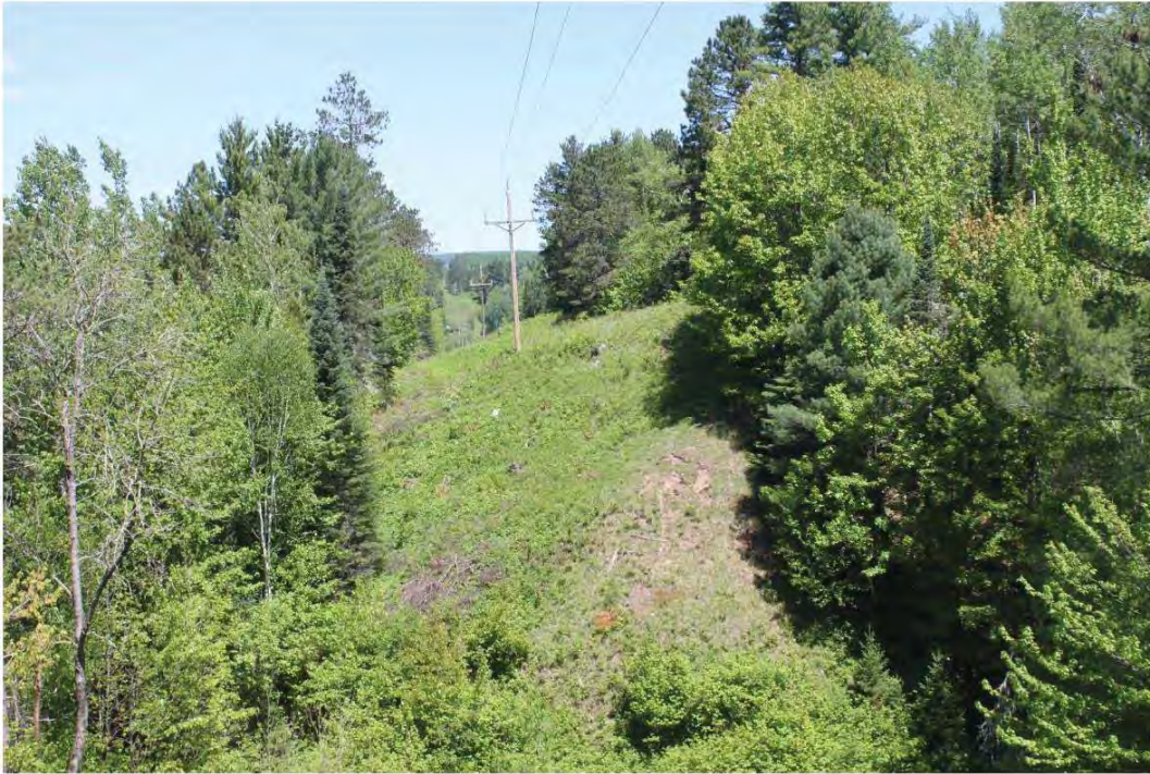
Figure 7. Photo of existing ROW where there is not a good location for an offset line.
