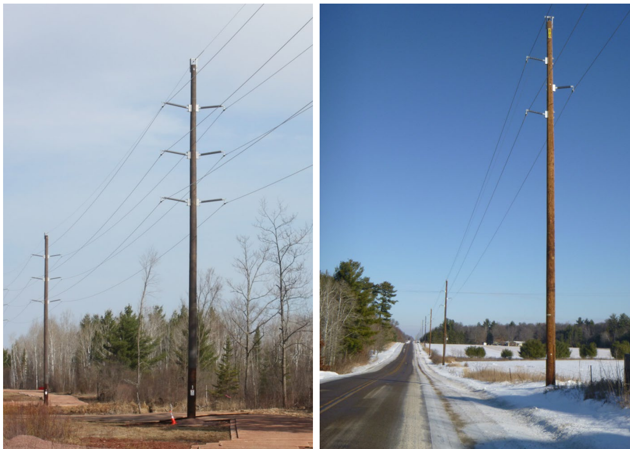
Figure 5.3-1 Typical Structure Types: Double-Circuit and Single-Circuit
