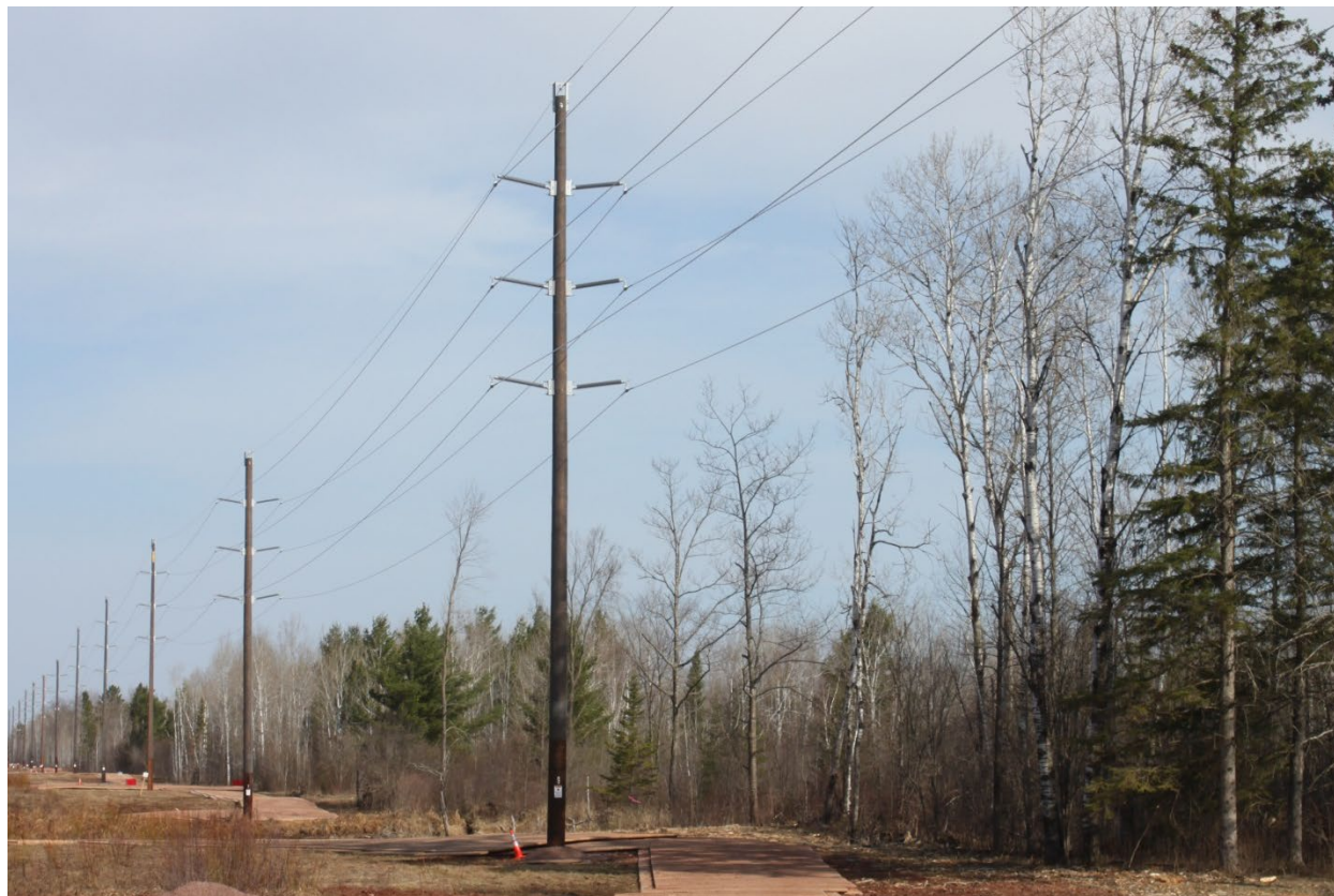
Figure 5.3-4 Typical Double-Circuit 34.5 kV/34.5 kV Structure Type
