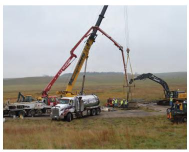
The last foundation is poured on the Big Stone South-Brookings County project. More than 33,000 cubic yards of concrete were used to construct project foundations.
