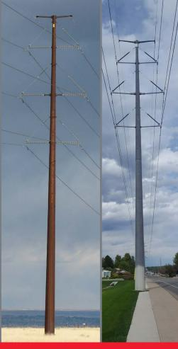
Construction on the Northern Colorado Area Plan includes using single-pole structures which will range between 80 and 130 feet in height.
