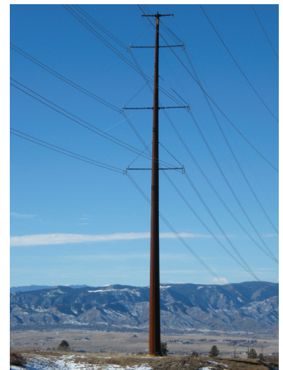
345 kV single pole, double circuit transmission structure
