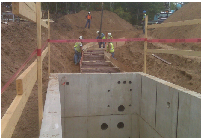
Crews work on an underground duct bank extending from a typical 8'x 8'x24' vault
