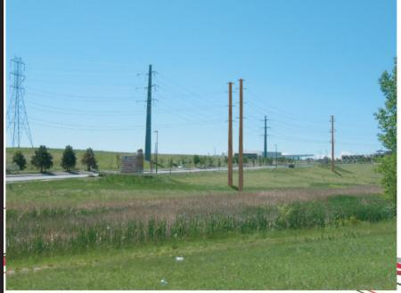
Self-Weathering Steel Structure Option
