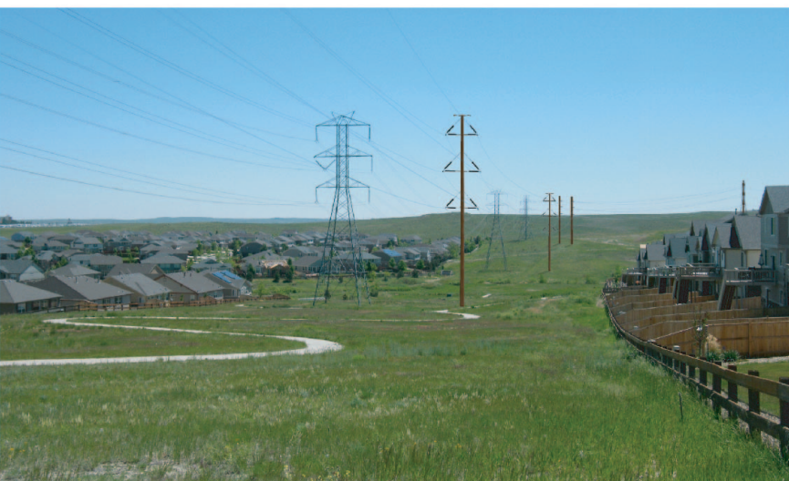
Self-Weathering Steel Structure Option
