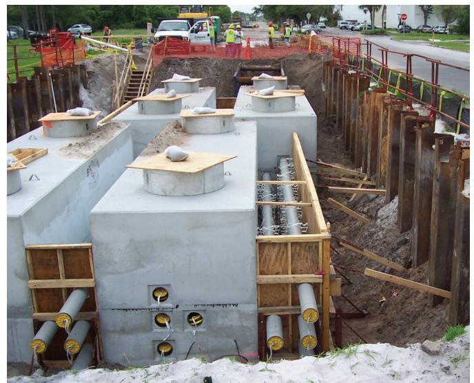
Underground transmission line construction
