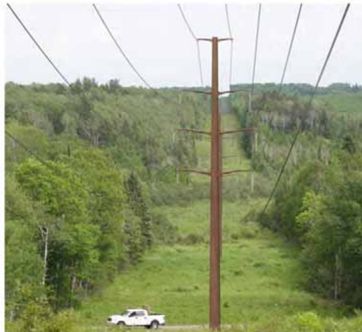
Proposed 161/69 kV Single Pole Weathering Steel Davit Arm Structures
