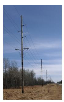
Single pole steel and wood structures approximately 50 to 60 feet in height are proposed on the Bayfield Second Circuit Project, with a 50–foot right–of–way. Some of the structures will require a distribution line be placed on the same structure.
