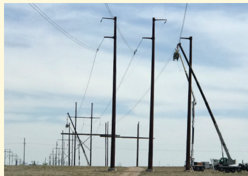
Crews finish stringing work on the Yoakum-Hobbs transmission line project near Hobbs, N.M.
