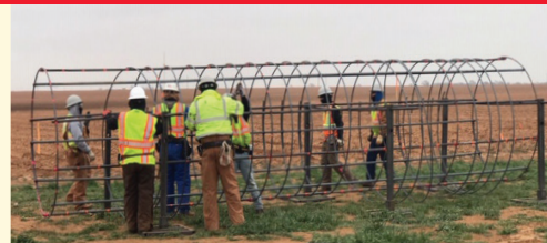
Crews build a rebar cage that will be used for a foundation on the final segment of the TUCO-Yoakum-Hobbs transmission line in Hale County, Texas.
