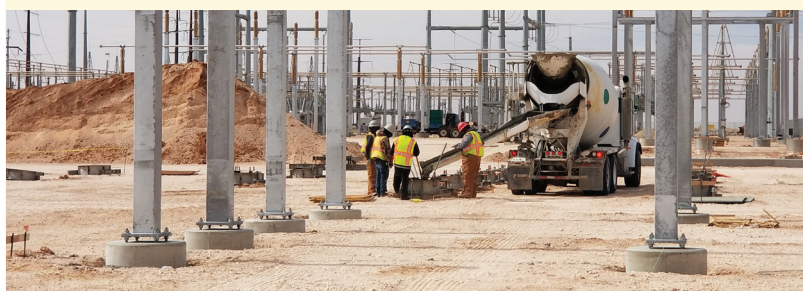
A foundation is poured for the Yoakum Substation expansion near Plains, Texas.
