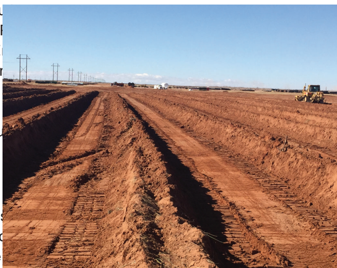
Grading is underway at the new Roadrunner substation site.
