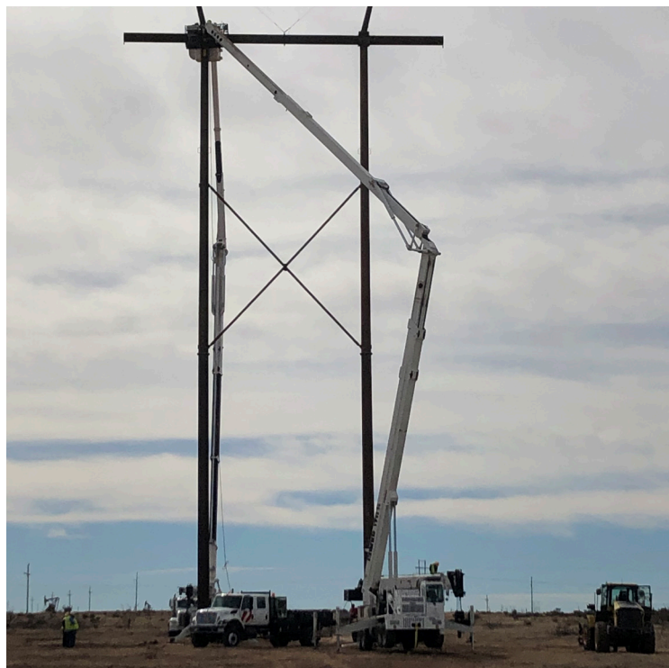
Crews set an h-frame steel structure in Eddy County, New Mexico.
