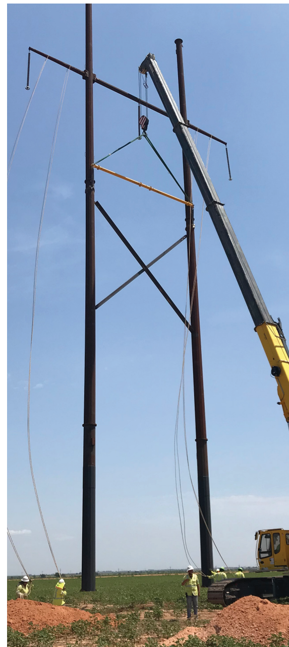
The last structure is set on the final segment of the TUCO-Yoakum-Hobbs transmission line. The final segment will be energized in June 2020.
