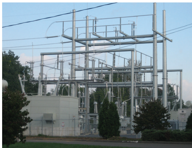
At either end of an underground section of the line, large one-acre transition structures (mini-substations) need to be constructed.
