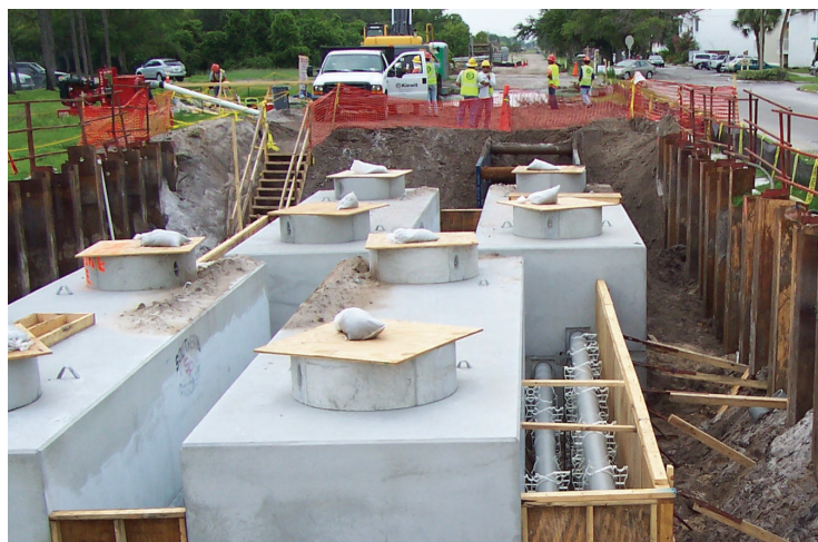
Garage-sized concrete access structures must be placed underground every 1,500 to 2,500 feet for maintenance and repair of an underground line.
